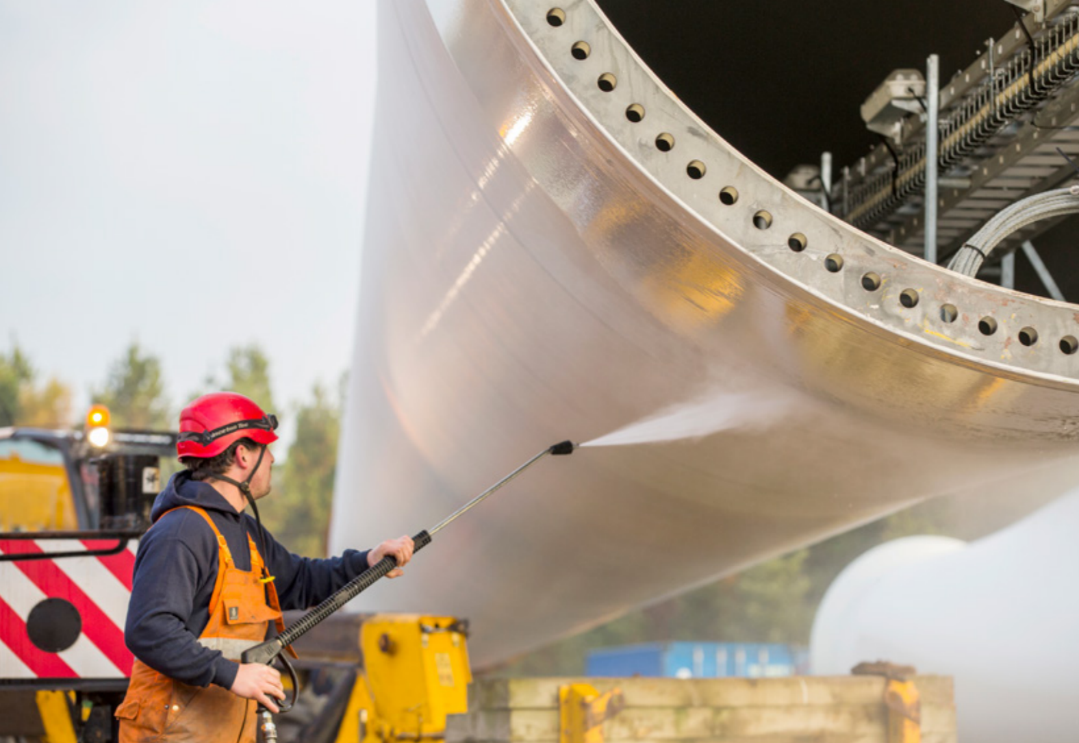
Turbine towers arrive in several parts and are constructed on site.
